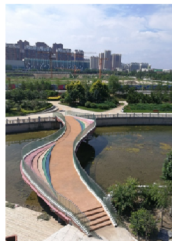
Figure 5. Aerial view of bridge
