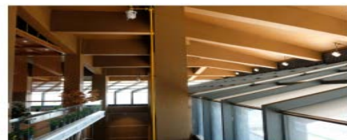
Figure 7. The cast-in-place reinforced concrete frame
