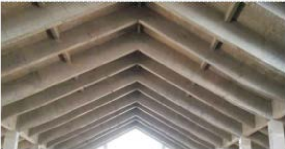
Figure 3. Cast-in-place appearance of roof beam
