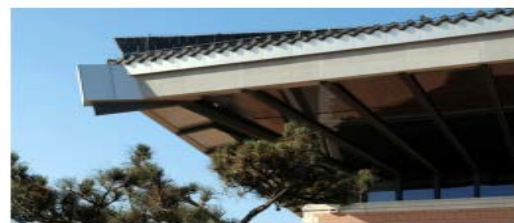
Figure 6. The cast-in-place reinforced concrete frame
