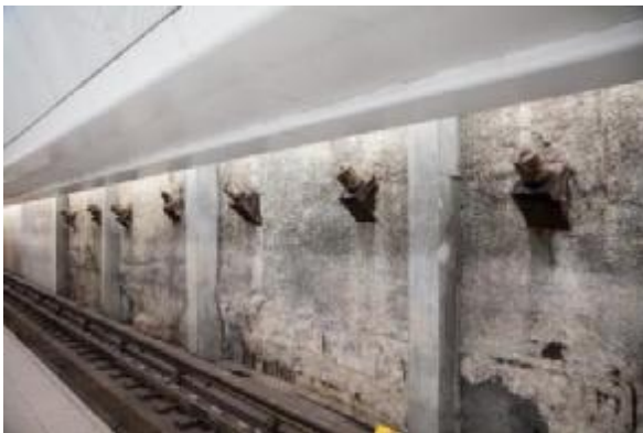
Figure 1. Original foundation wall in new station
