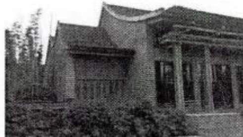
Figure 10. Roof overhanging eaves of Lanxi court
