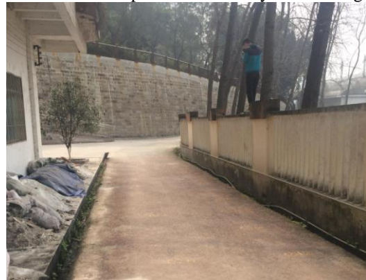
Figure 3. Initial condition of road
