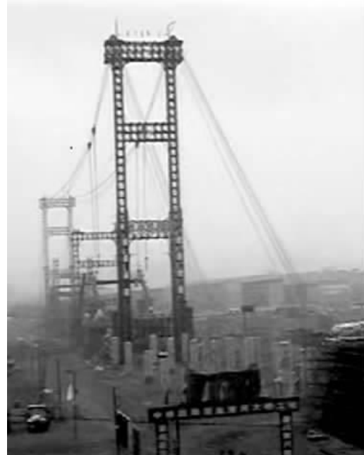
Figure 2. The overall arrangement of tower
