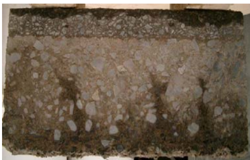
Figure 3. Fatigue Cracking in CSL Trenching (Moisture in Cracks) (Yeo 2008)
