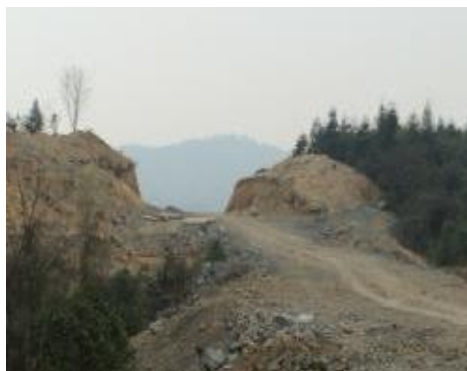
Figure 2. Mountain excavation face
