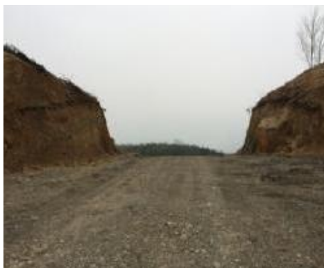
Figure 3. Mountain excavation face 2
