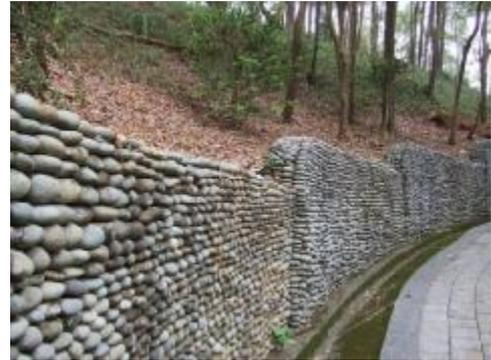
Figure 3. Cobblestone retaining wall
