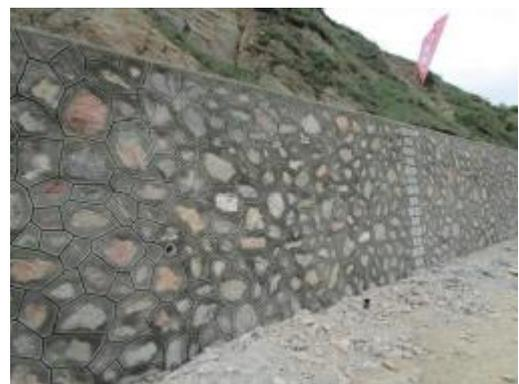
Figure 14. Ordinary stone retaining wall
